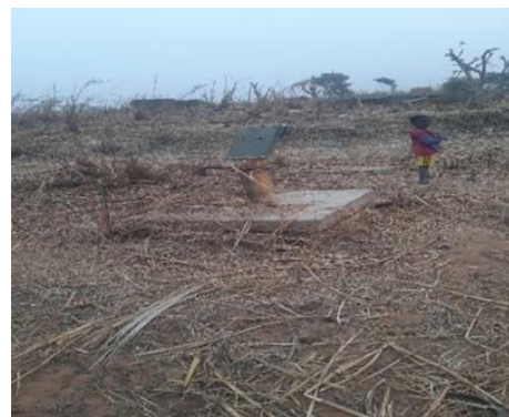
Figure.3 Abandoned fountain hydrant
